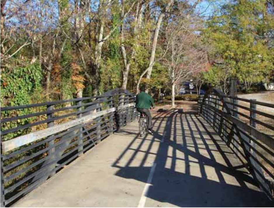
Bike bridge in Atlanta, Georgia (Photo: VHB).
