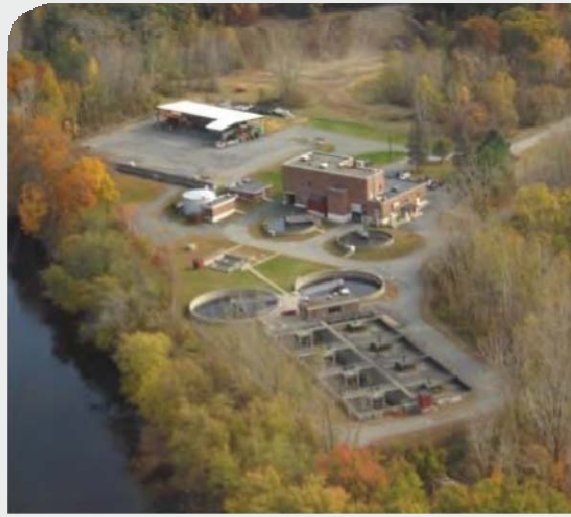
wastewater treatment facility
